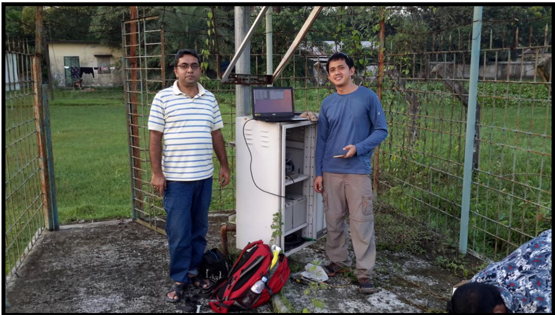
Photo: Manual data downloading process in Haluaghat station.
